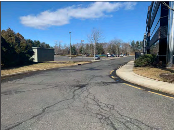
Figure 15: Cracking of asphalt in parking lot.
