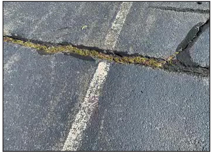
Figure 18: Cracking of asphalt within parking lot.
