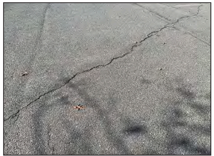
Figure 10: Cracking of asphalt in parking lot.
