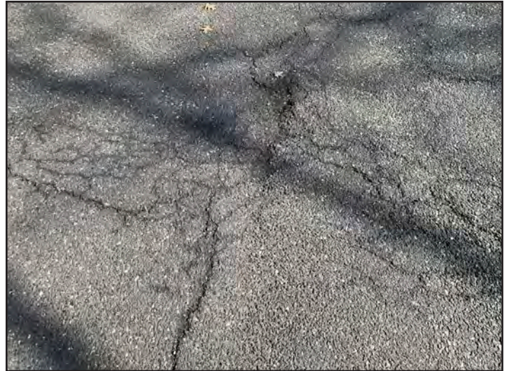
Figure 8: Cracking of asphalt in parking lot.
