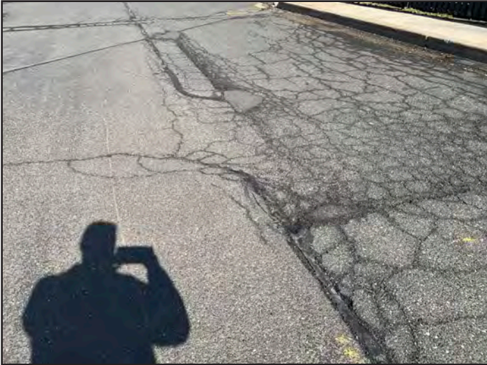
Figure 13: Cracking of asphalt in parking lot.
