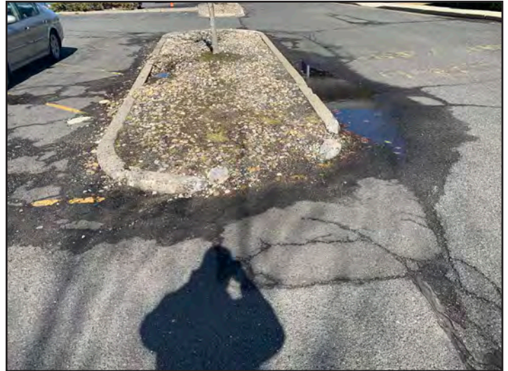
Figure 14: Parking island in poor condition and cracking of asphalt
