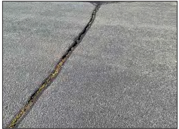
Figure 18: Cracking of asphalt and fading of striping parking spaces within parking lot.
