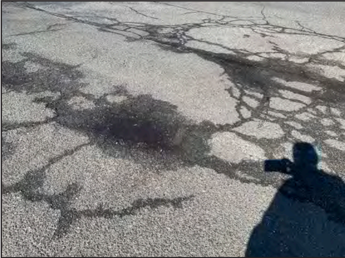
Figure 13: Cracking of asphalt in parking lot.
