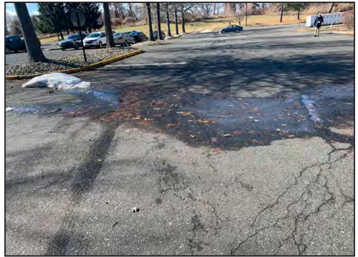
Figure 12: Cracking of the parking asphalt.
