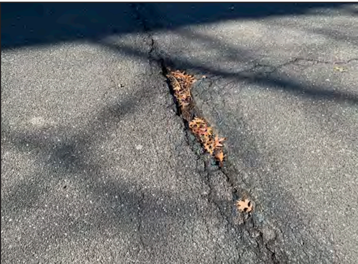
Figure 11: Cracking of parking asphalt.
