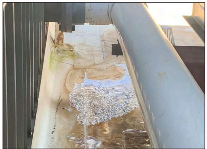
Figure 12: Water retention on the roof due to inadequate drainage design.
