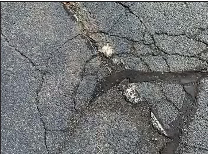
Figure 17: Cracking of asphalt and fading of striping parking spaces within parking lot.
