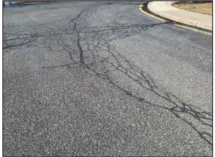
Figure 14: Cracking of asphalt in parking lot.
