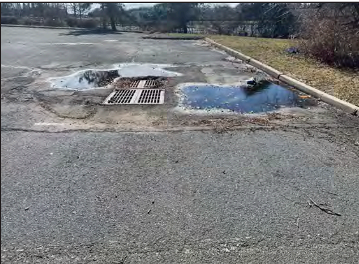
Figure 17: Water retention in parking lot due to limited stormwater management.
