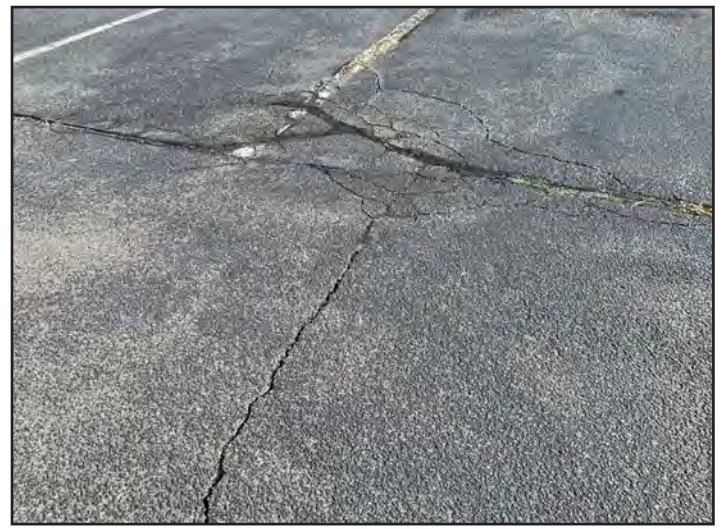
Figure 16: Cracking of asphalt and fading of striping parking spaces within parking lot.
