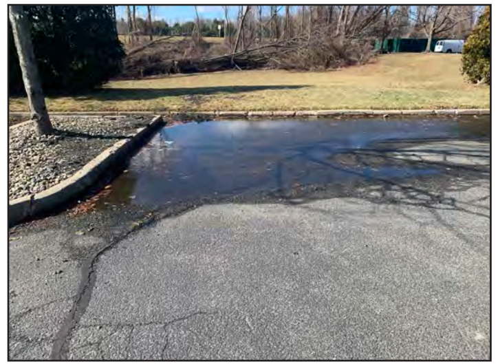
Figure 16: Water retention in parking lot due to limited stormwater management.
