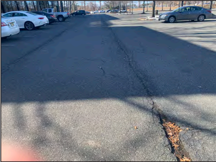
Figure 7: Cracking of asphalt in parking lot.
