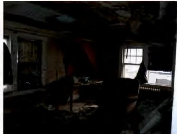
A view of the second floor apartment of the Lunney's building. Seen here is piled trash and debris, a leaking roof and deteriorated ceiling, broken and taped windows, and deteriorated wall coverings. The building represents unwholesome living and working conditions in its current condition.
