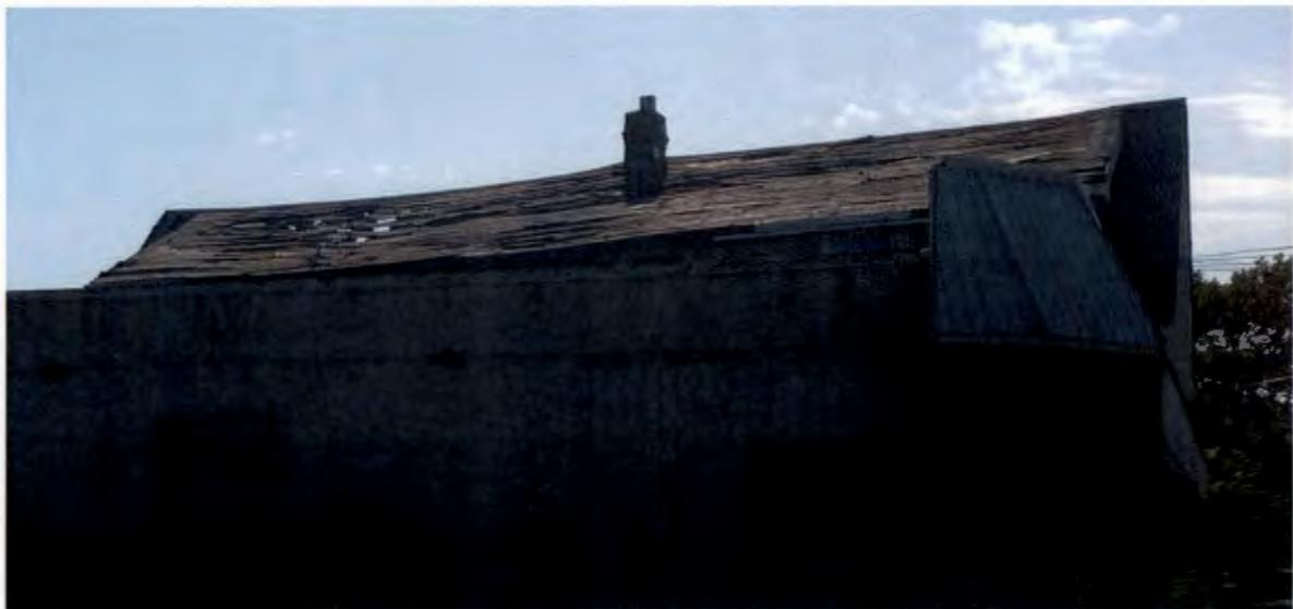
A second photo of the existing condition of the roof of the existing Lunney's building. The roof is partially collapsed.
