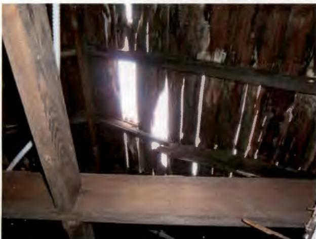
A view of the roof of the Lunney's building. The roof exhibits rotting wood, significant holes, and missing shingles, plywood sheathing, and felt underlayment.
