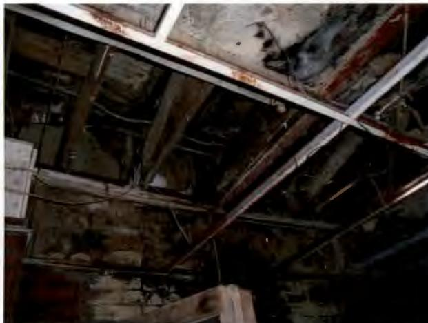
A second photo of the first floor ceiling of Lunney's. Depicted here are exposed water pipes, missing ceiling tiles, and rusting drop ceiling framework. *(Photo courtesy of Middletown Township)*
