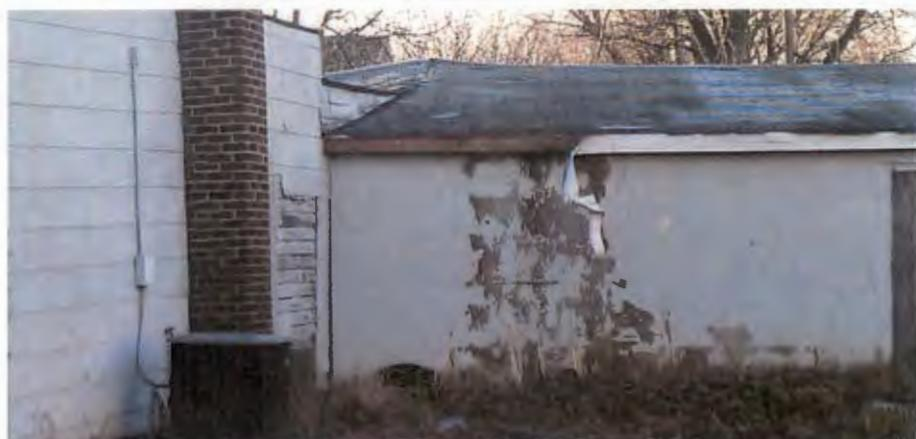
A view of the west side of the existing Lunney's building on Block 70, Lots 2 and 3. The exterior walls of the building exhibit peeling paint and overall lack of maintenance. In addition, the roof is dilapidated and partially collapsed. The roof section seen here exhibits deteriorated and detached fascia, missing roof shingles and bowing.
