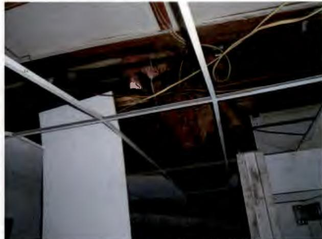
View of the first floor ceiling of the Lunney's building. This photo depicts exposed insulation and wiring and missing ceiling tiles due to overall neglect. The building's interior is dilapidated and represents unwholesome working conditions, and the building is untenantable in its current state. *(Photo courtesy of Middletown Township)*
