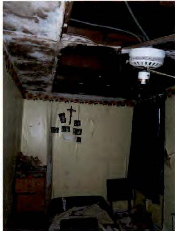
Bedroom area of the second floor apartment in the Lunney's building. Significant portions of the ceiling are missing, exposing the roof structure of the building. There is debris throughout the building, and the building is uninhabitable in its current state.
