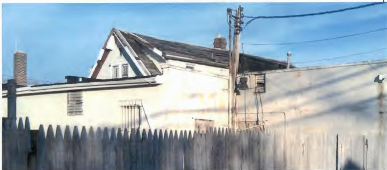
View of the existing Lunney's building from Ocean Avenue, looking northwest. The use of the existing building has been discontinued and the building now exhibits signs of dilapidation. This photo depicts peeling and missing exterior paint, boarded up windows, haphazardly organized wiring and damaged exterior ventilation grilles. The roof section seen here exhibits significant deterioration including deteriorating fascia and soffits and swaths of missing shingles.
