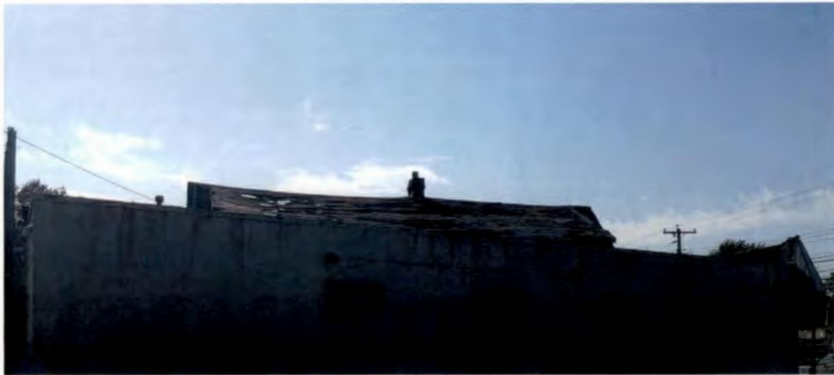
A view of the eastern portion of the roof of the Lunney's building, Block 70, Lots 2 and 3. The building exhibits significant signs of dilapidation. Many of the shingles on the existing roof are missing revealing the plywood sheathing and felt underlayment of the existing roof. In other areas, the roof is completely rotted and partially collapsed.
