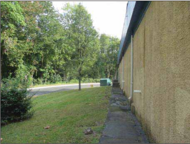
Image 13: Water damage along asphalt sidewalk at rear of the building with erosion.
