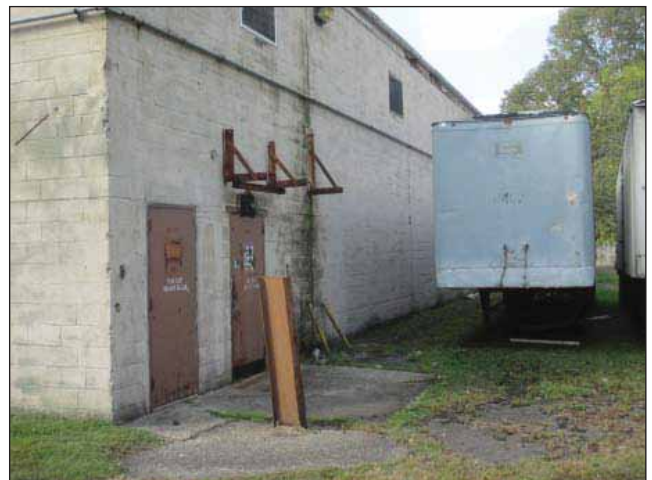
Image 23: Rear elevation with water damage along drain pipe.
