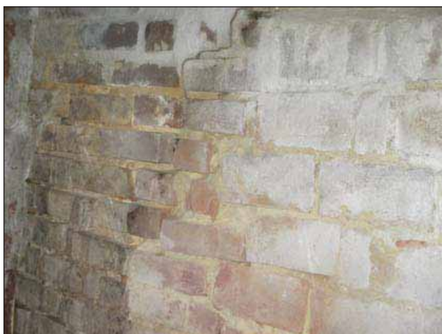
Image 17: Cracking and bowing in basement foundation wall.
