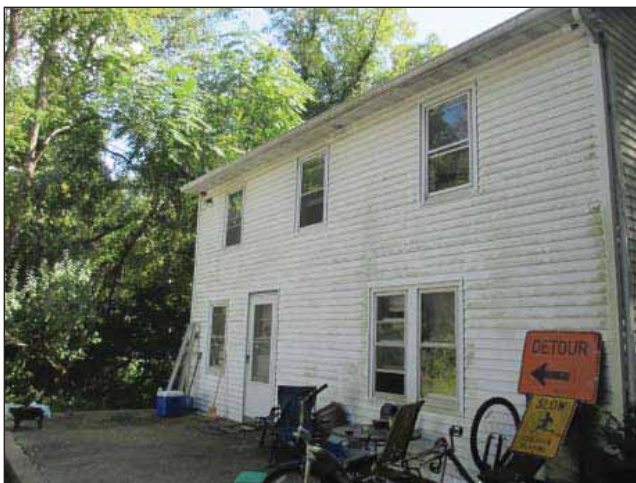
Image 5: Rear facade with mold and mildew on siding.
