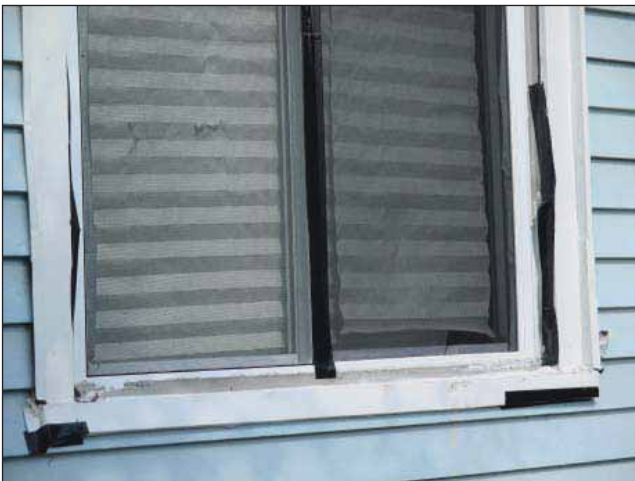
Image 15: Damage along existing window frames.
