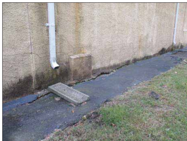
Image 8: Water damage along asphalt sidewalk at rear of the building with erosion.
