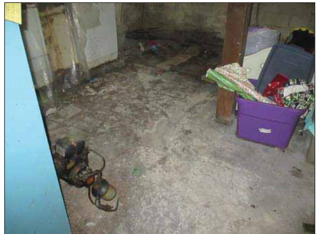
Image 6: Remnants of water on basement floor with wet conditions all the exterior perimeter walls.
