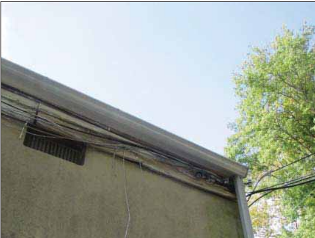
Image 15: Water damage and rotting along rear roof line.
