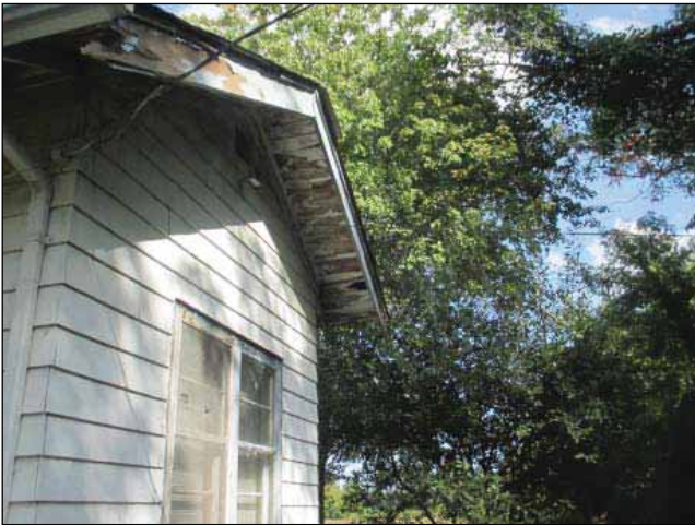
Image 5: Degraded roof beams.
