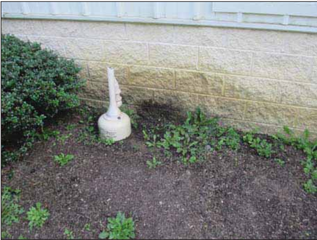
Image 13: Water damage at the front base of the building caused by a lack of proper drainage
