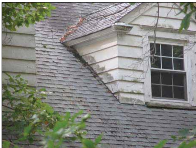
Image 12: Damage to the roof and eaves at the rear of the building.
