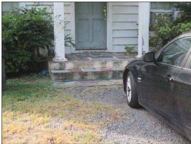
Image 10: Damage to front stoop and pillars of two story residential building.
