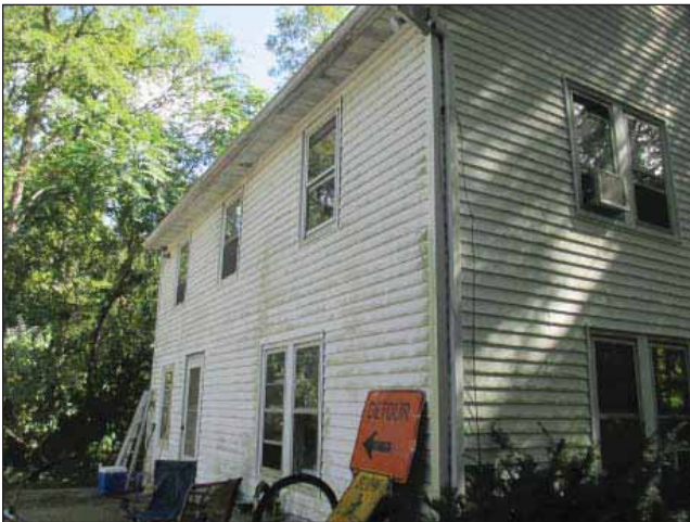
Image 3: Rear facade with mold and mildew on siding.
