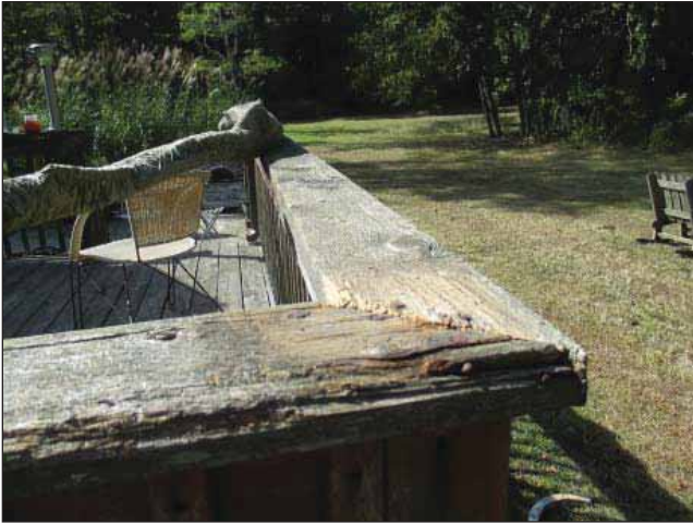
Image 7: Rear porch with rotting wood and deterioration.
