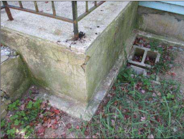
Image 7: Rear steps with corroded and broken concrete steps.
