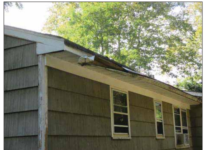
Image 6: Significant damage / rotting to the existing roof and gutters.
