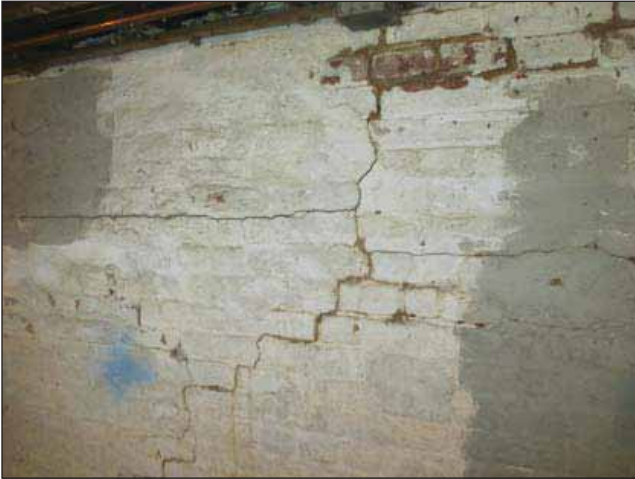
Image 19: Crack in foundation wall in the basement.
