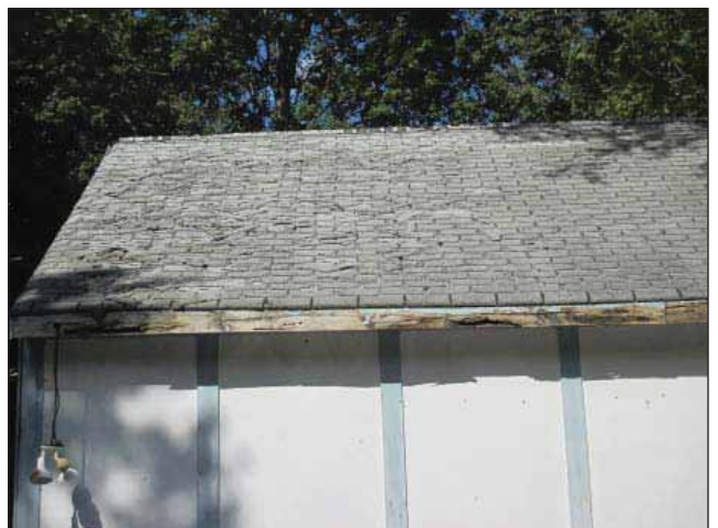
Image 12: Rooting wood along roof line.
