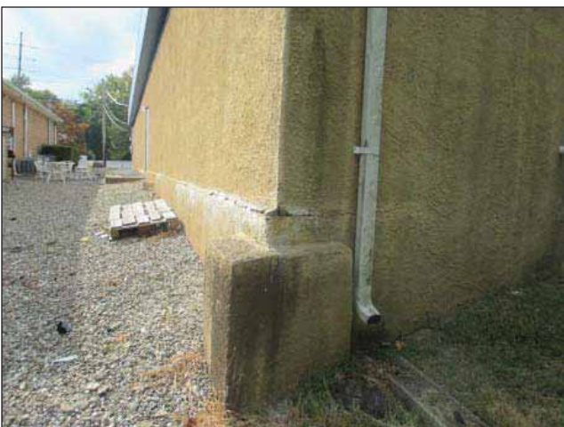
Image 5: Water damage along rear base of building with cracking in efface.
