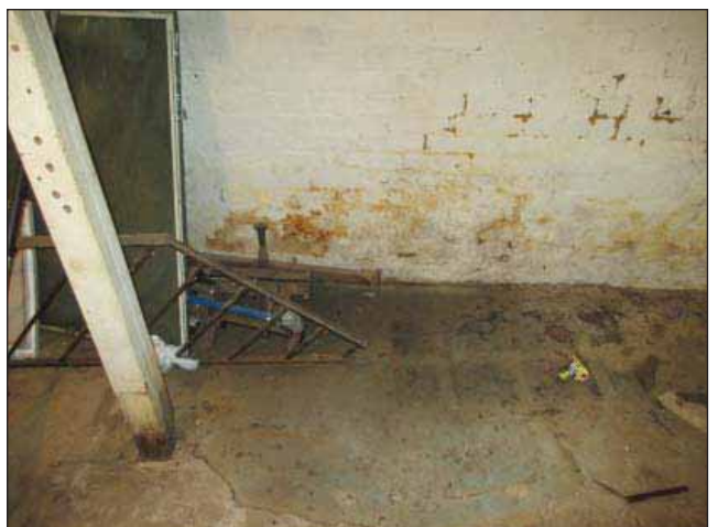
Image 18: Basement with water stains.
