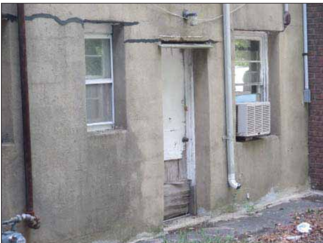
Image 11: Rear wall with cracking and repairs. Downspouts directly onto the rear drive.
