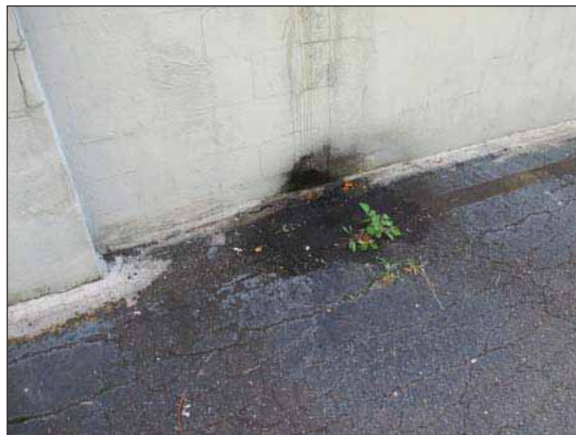
Image 22: Water damage at the rear base of the building.
