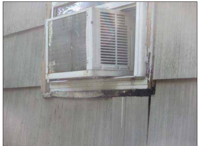
Image 16: Rotting wood framing around air conditioning unit.
