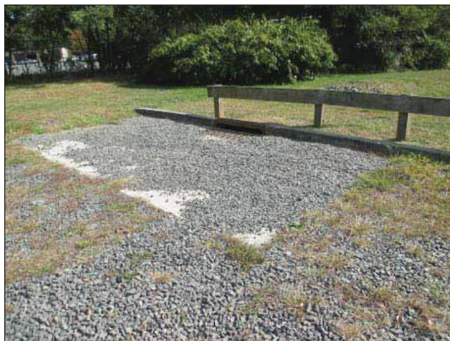
Image 8: Western drain inlet with significant gravel surrounding the inlet
