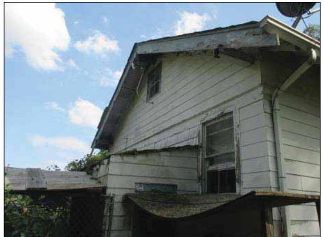
Image 7: Collapsing rear room with damage to roof beams.
