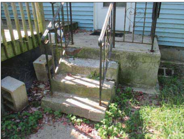
Image 5: Rear steps with corroded and broken concrete steps.
