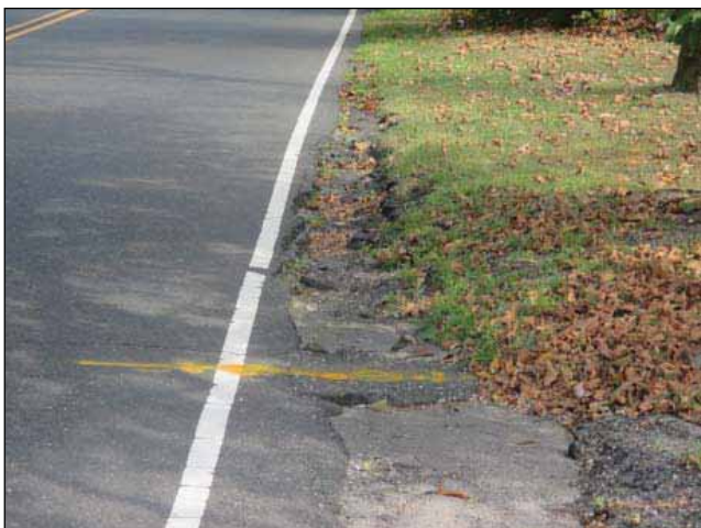
Image 2: Erosion along Kings Highway with no curb and gutter
