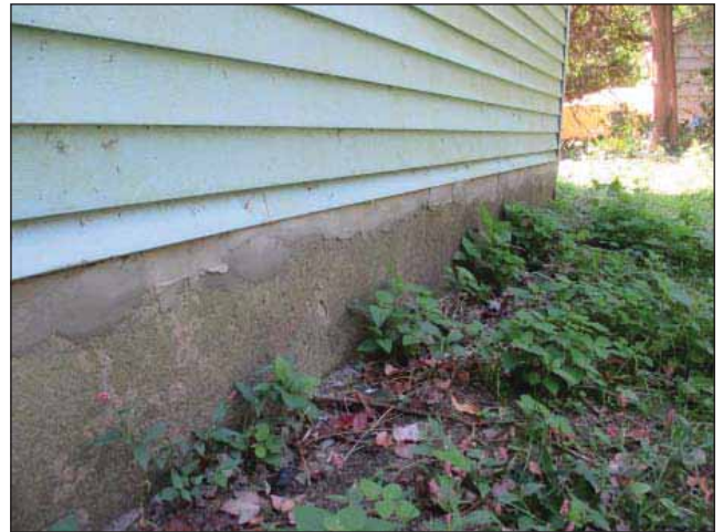
Image 8: Patching along base of single family house
