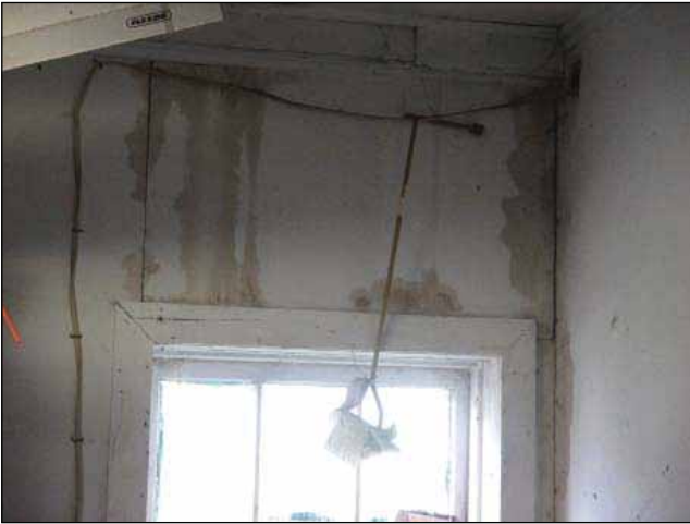
Image 40: Water damage along interior wall in barn structure.
