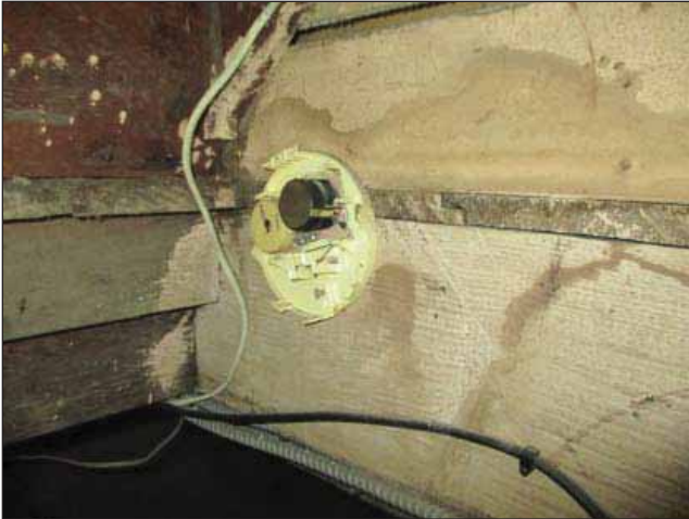
Image 19: Electrical lines and cracks in foundation walls.
