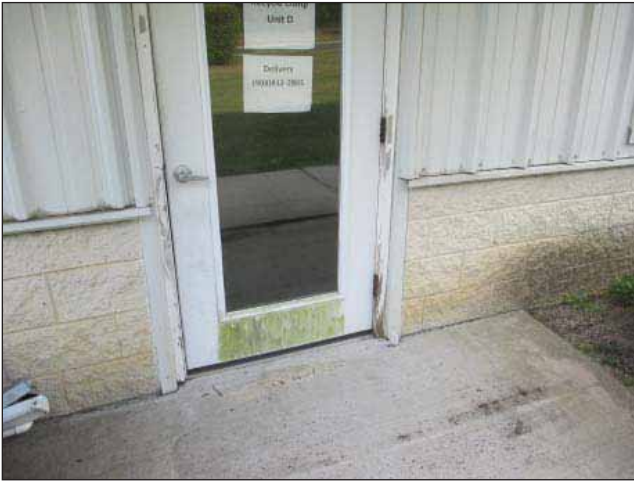
Image 19: Water damage and signs of mold at the base of the building entrance
