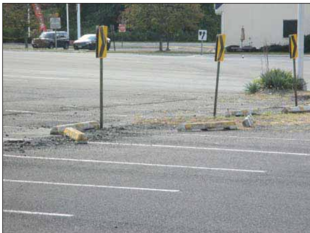
Image 40: Erosion of existing parking area depicting run-off damage toward Route 35.
