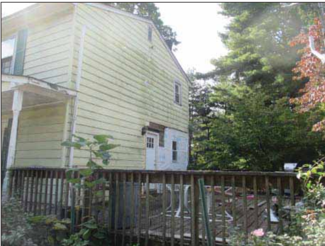
Image 3: Back porch with rotting wood on porch fascia and rear portion of siding missing.
