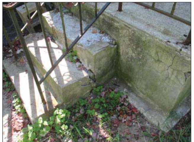
Image 6: Rear steps with corroded and broken concrete steps.
