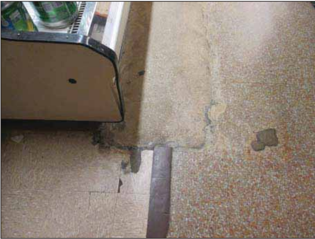
Image 8: Water damage and repair on the retail store floor.
