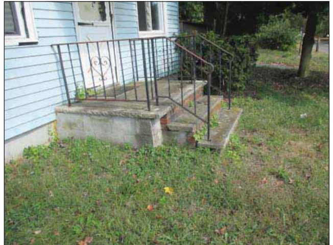
Image 14: Damage along front steps. Missing walk to the driveway or Kanes Lane.
