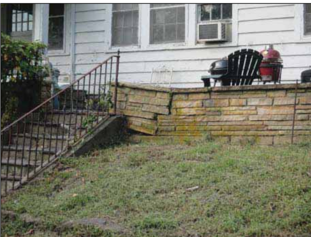
Image 2: Rear yard retaining wall collapsing
