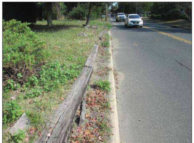
Image 16: Retaining wall along Kanes Road that is leaning toward the street and is damaged and rotting.
