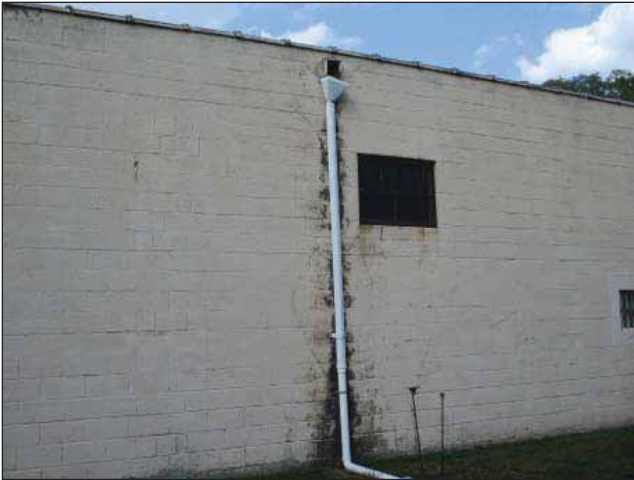
Image 20: Water damage along drain pipe area on side elevation.
