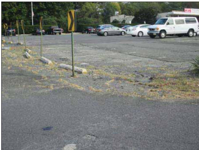
Image 41: Erosion of existing parking area depicting run-off damage toward Route 35.
