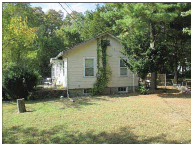
Image 10: Side of house with vegetation growing up the side into the attic space.
