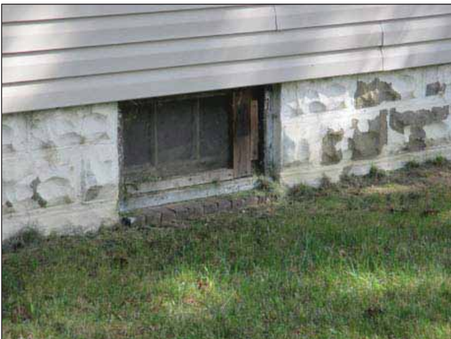
Image 11: Basement window with rotting wood on frame.
