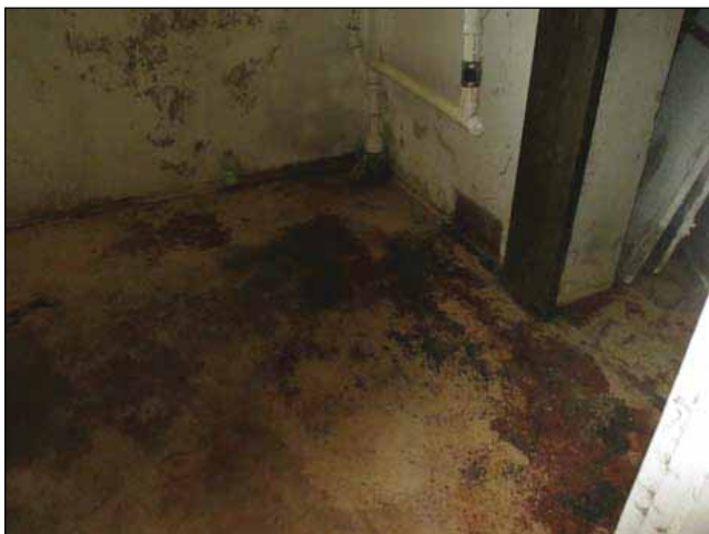
Image 24: Basement floor with water damage.
