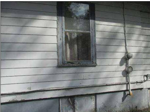
Image 6: Rotting wood framing at windows.
