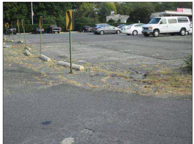
Image 12: Erosion of existing parking area depicting run-off damage toward Route 35.
