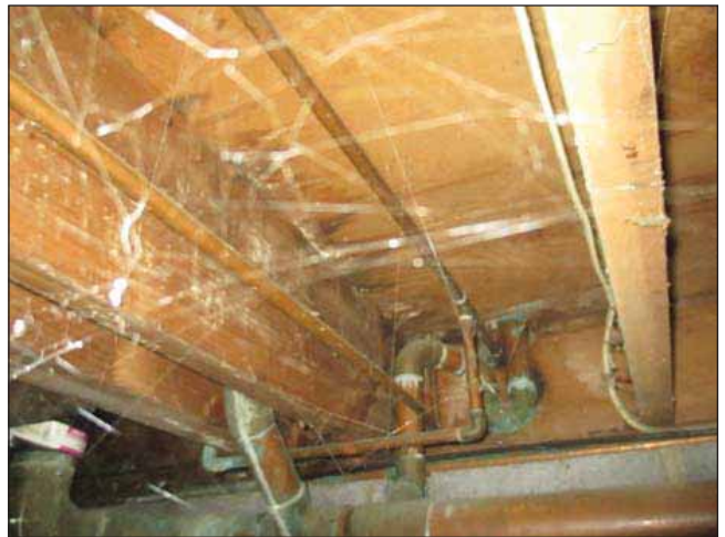
Image 20: Basement with discoloration of work indicating water damage.
