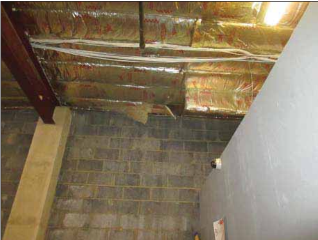
Image 16: Leaching along storage area walls depicting water damage.
