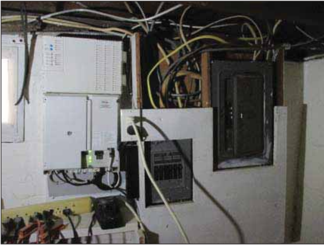
Image 13: Exposed wiring in basement.
