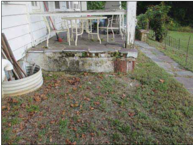
Image 22: Rear port with damage to concrete.
