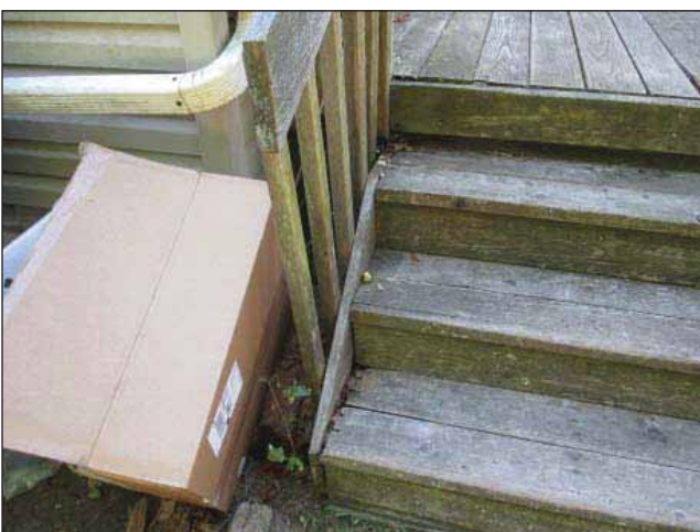
Image 5: Rear porch with rotting wood and deterioration.
