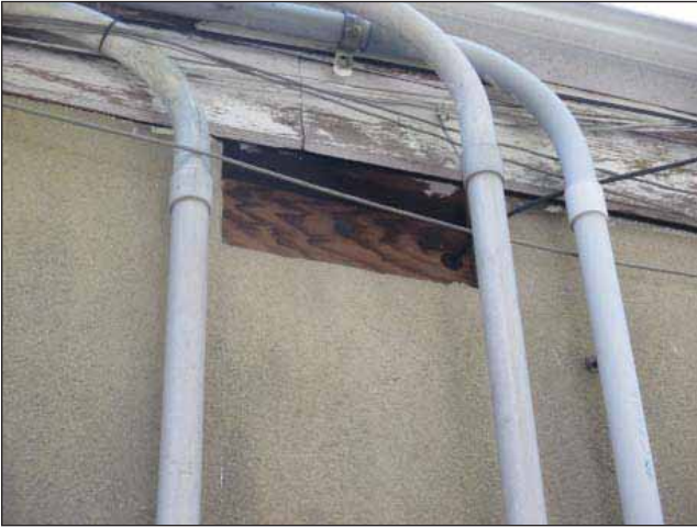
Image 13: Patch of hole in rear part of the building with wood.
