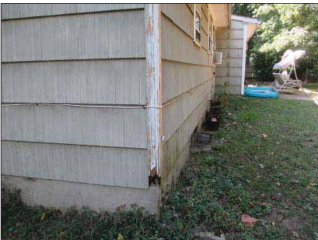
Image 5: Rotting wood along side of rear and side facade.
