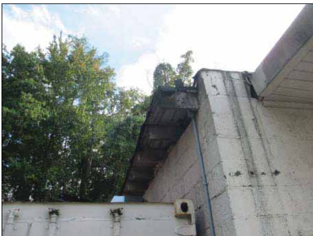
Image 2: Roof with rotting beams.
