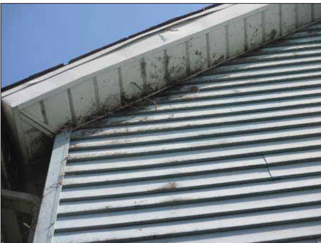
Image 11: Damage from previous plant materials on side of house.
