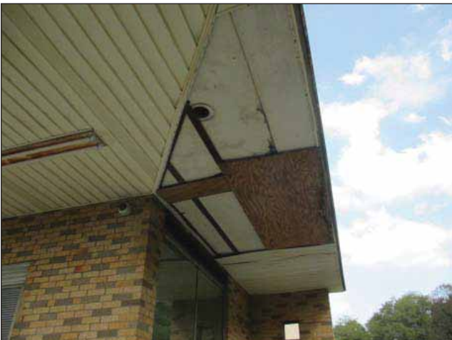
Image 18: Exterior overhang with missing ceiling panels.
