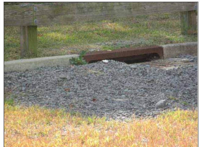
Image 6: Eastern drain inlet at the rear parking area with significant gravel around the inlet
