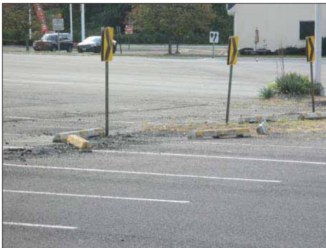
Image 11: Erosion of existing parking area depicting run-off damage toward Route 35.
