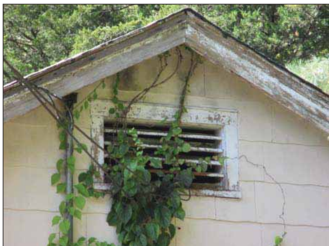
Image 11: Side of house with vegetation growing up the side into the attic space.
