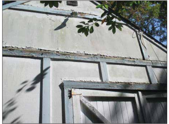
Image 8: Deterioration of side panels at barn.
