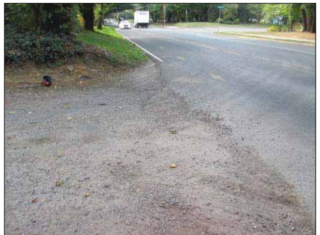
Image 9: Driveway entrance depicting a lack of sidewalks and drainage from the driveway into the road.
