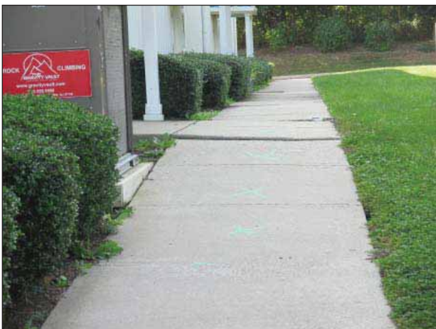
Image 9: Front entrance with sidewalk heaving.
