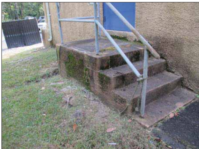
Image 9: Rear stairs with erosion caused by water run-off from roof.
