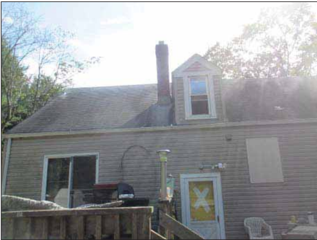
Image 9: Multiple rear door and window patched with wood paneling.
