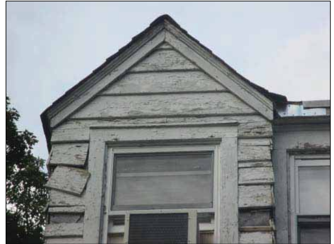
Image 19: Boards falling off and missing from rear eave.
