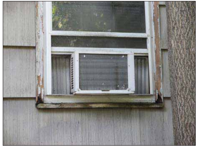
Image 2: Rotting wood along window frame.
