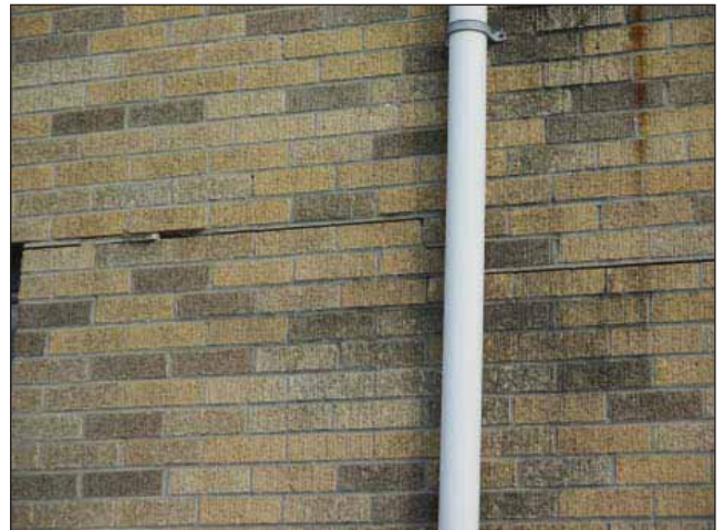
Image 7: Separation of bricks along building facade.
