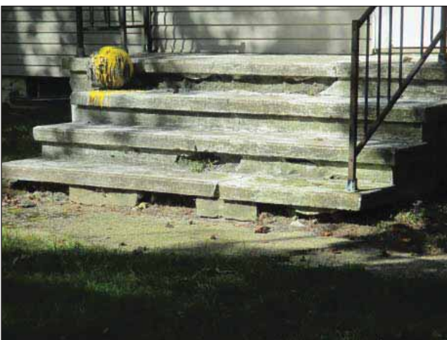
Image 3: Front steps damaged and cracked.
