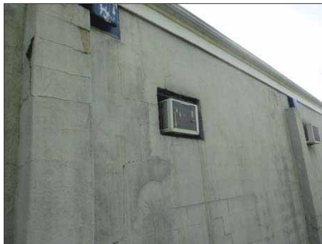
Image 20: Cracking and peeling of facade along rear wall of building.
