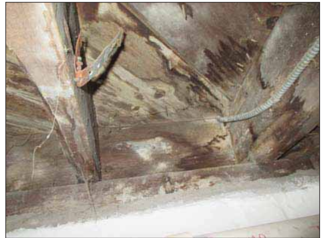
Image 16: Rotting wood and water damage in basement.
