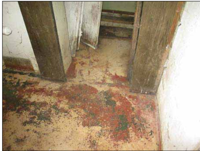
Image 23: Basement floor with water damage.
