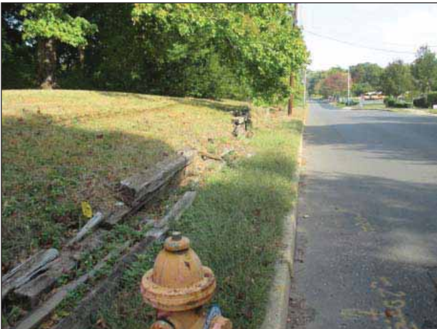
Image 5: Wood tie retaining wall on Kanes Lane without any sidewalk that is rotting and leaning toward the road.
