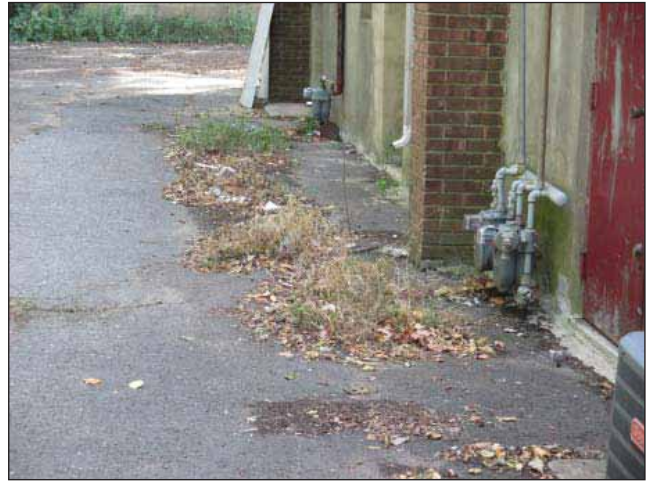
Image 14: Roof drains directly onto the asphalt area.
