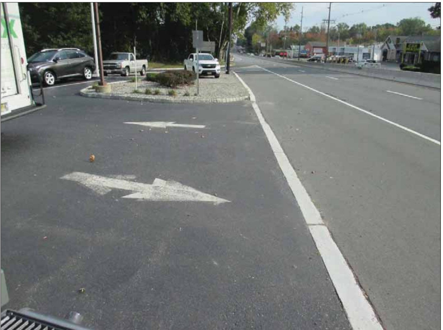
Image 1: Entrance off Highway 35 with FedEx truck parked in exiting lane. Vehicles are parked in the median which creates site line issues entering and exiting the parking lot.
