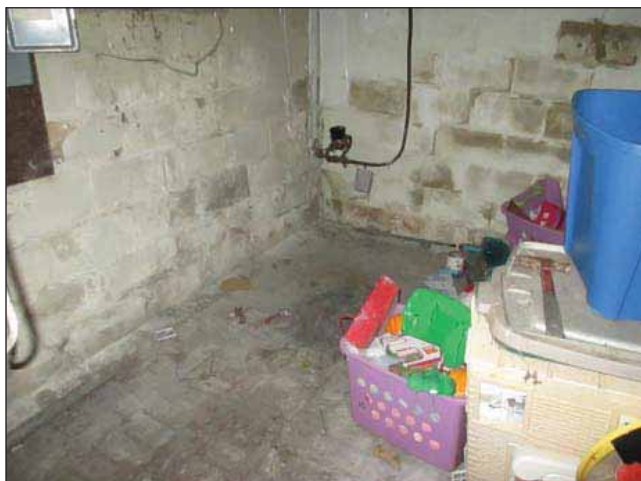
Image 9: Water damage and cracking along exterior basement wall.
