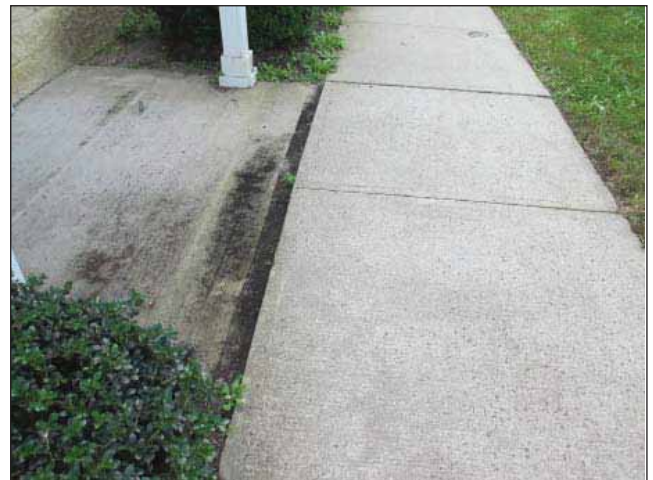
Image 18: Damage at the sidewalk and entrance pad caused by a lack of proper drainage
