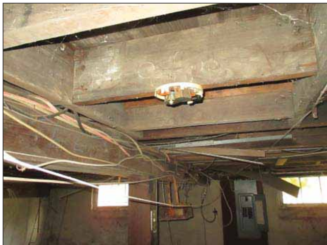
Image 7: Exposed and hanging wiring in basement with missing fire alarm.
