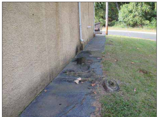
Image 6: Water damage along asphalt sidewalk at rear of the building with erosion.
