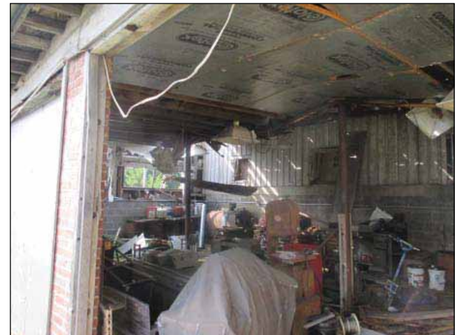
Image 43: Collapsing roof of barn structure side.
