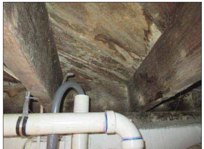
Image 18: Water damage on basement ceiling.
