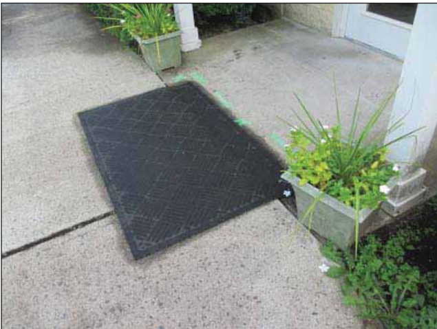
Image 15: Mat at entrance to cover water damage that cracked entrance step caused by water damage
