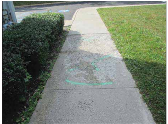
Image 20: Deterioration of the sidewalk caused by water damage
