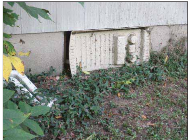
Image 4: Temporary plastic covering over opening to basement.
