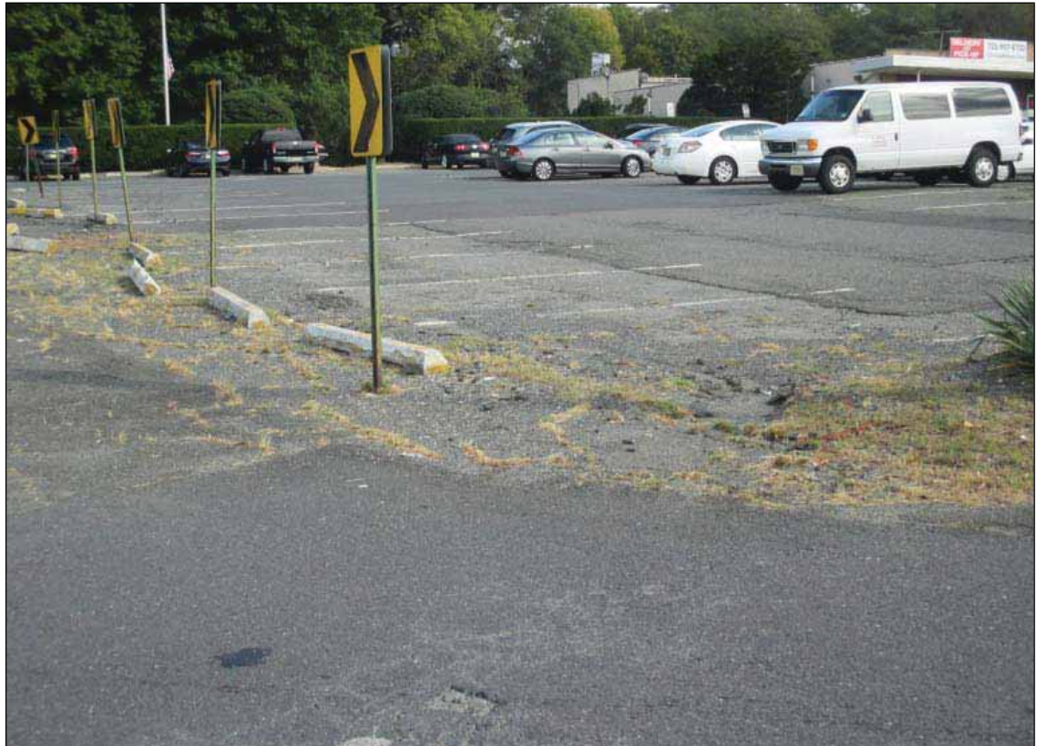
Image 1: Erosion of existing parking area depicting run-off damage toward Route 35.
