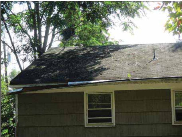
Image 15: Damage to rear roof with rotting fascia boards and moss on the roof.
