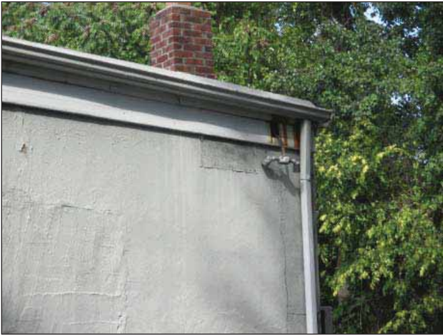
Image 7: South wall with water damage.
