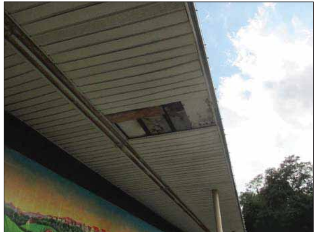
Image 17: Exterior overhang with missing ceiling panels
