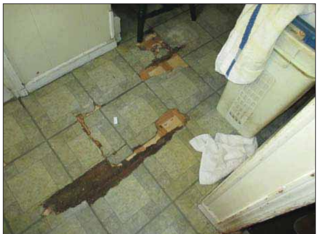
Image 18: Water damage in back entry.
