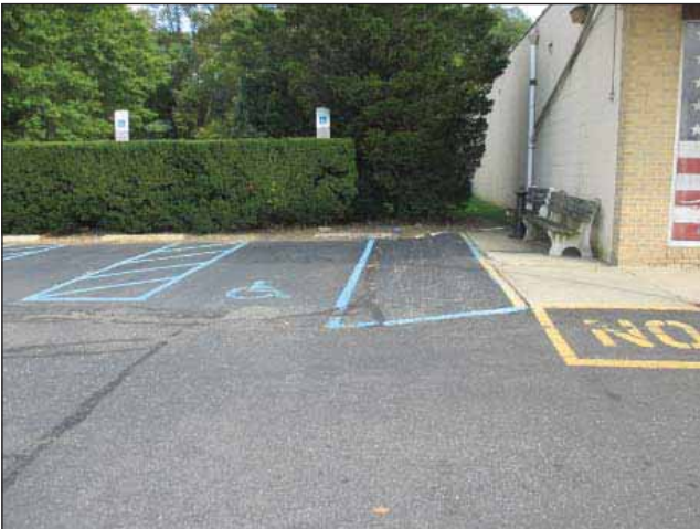
Image 32: Handicap spaces on side of the building with no striping.
