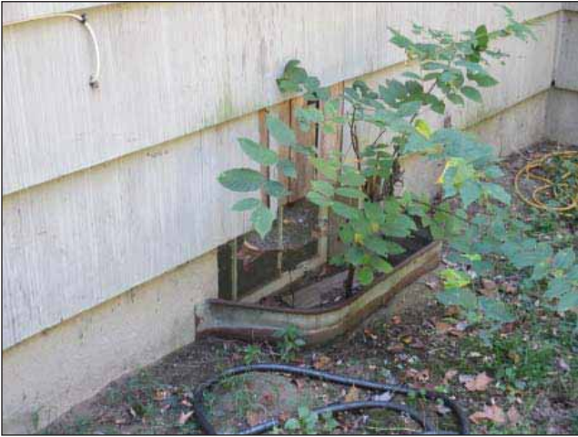
Image 7: Damage to the siding along rear facade.
