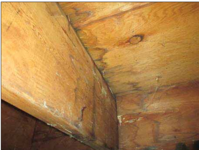
Image 23: Beams in basement with water damage.
