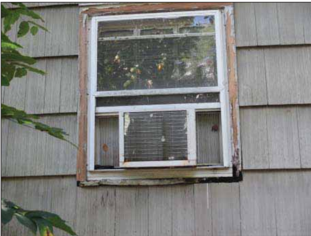
Image 3: Rotting wood along window frame.
