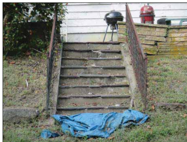
Image 15: Rear steps and retaining wall collapse
