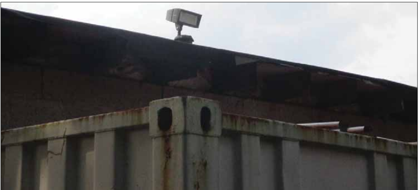
Image 1: Exposed insulation, water damage to beams and concrete with rusting
