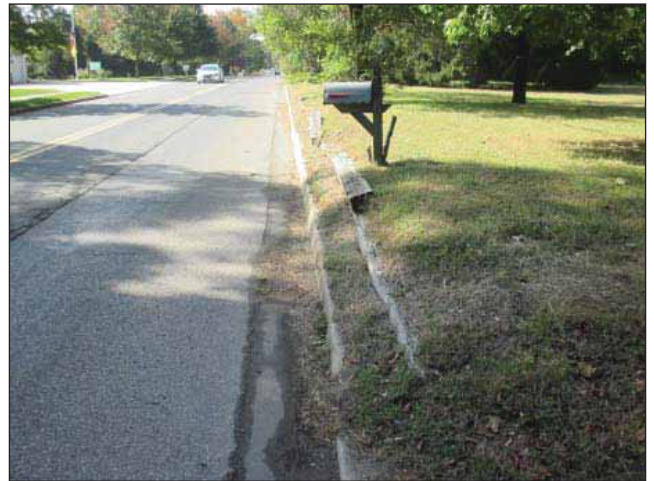
Image 2: Wood tie retaining wall on Kanes Lane leaning toward the street with no sidewalk.
