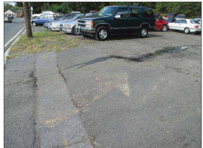
Image 9: Grades along front entrance going from the property to Highway 35 without any storm water management controls.
