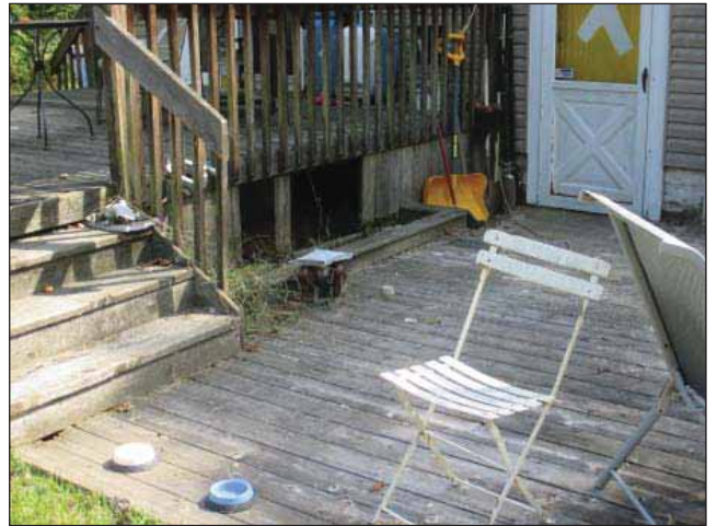
Image 10: Rear at grade porch with rotting wood and wood panel on rear door.
