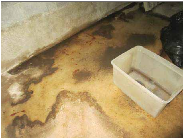
Image 21: Standing water and discoloration of floor.
