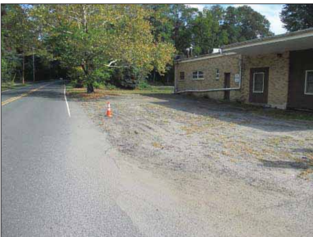
Image 8: Side view of building with asphalt and gravel depicting erosion caused by storm water run off along Kings Highway East.
