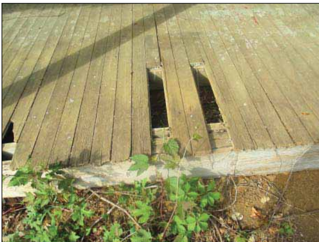
Image 53: Slats of cabin porch missing / broken.
