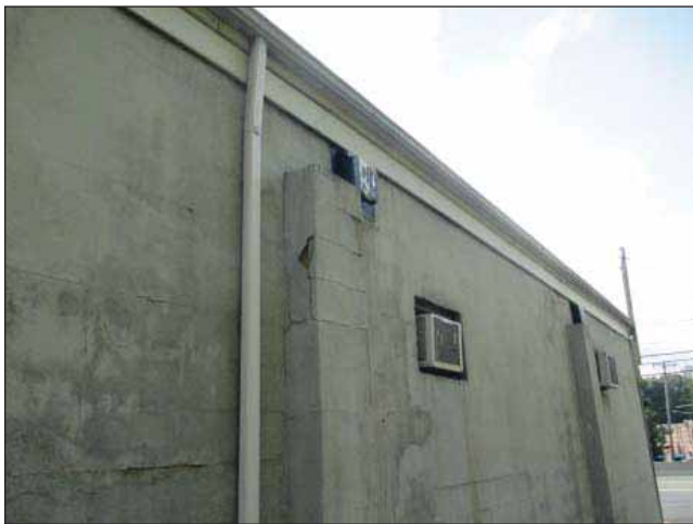
Image 19: Cracking and peeling of facade along rear wall of building.
