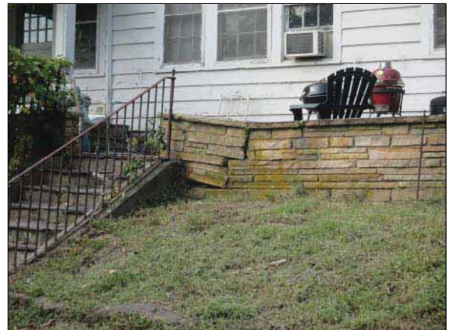
Image 21: Rear yard retaining wall collapsing
