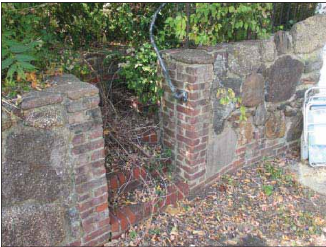
Image 3: Overgrowth of vegetation at steps to rear with concrete patching over areas.
