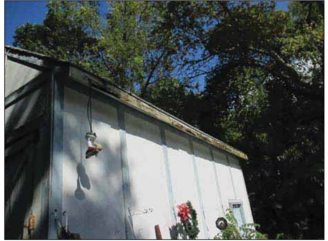
Image 10: Degradation of roof at barn.
