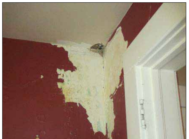
Image 33: Cracking in main house with water damage.
