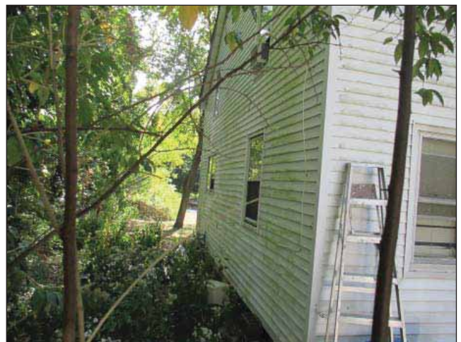
Image 6: Side facade with mold and mildew on siding.
