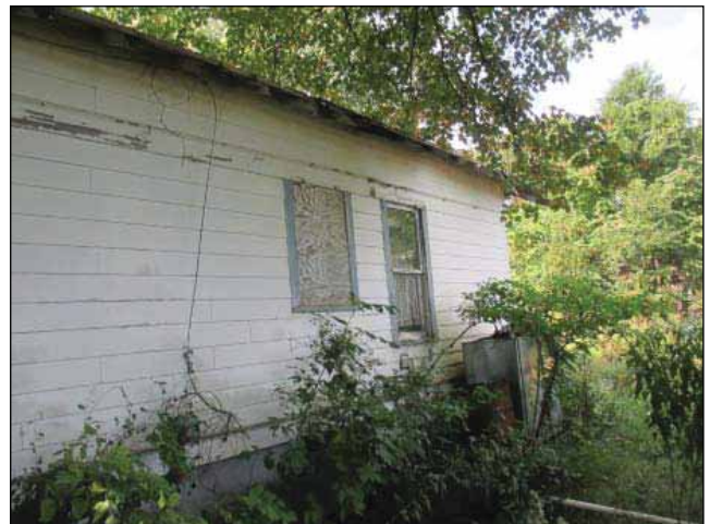
Image 11: Roof completely deteriorated at rear of house with window boarded up.
