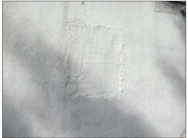
Image 8: Patch work of exterior wall.
