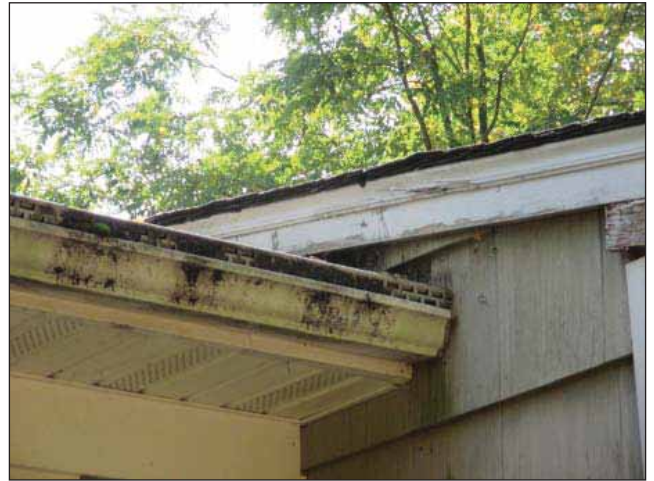
Image 8: Rotting and decay along roof line convergence.
