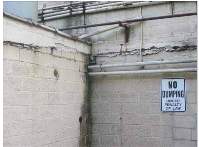
Image 27: Rear elevation depicting water damage along joint between buildings.
