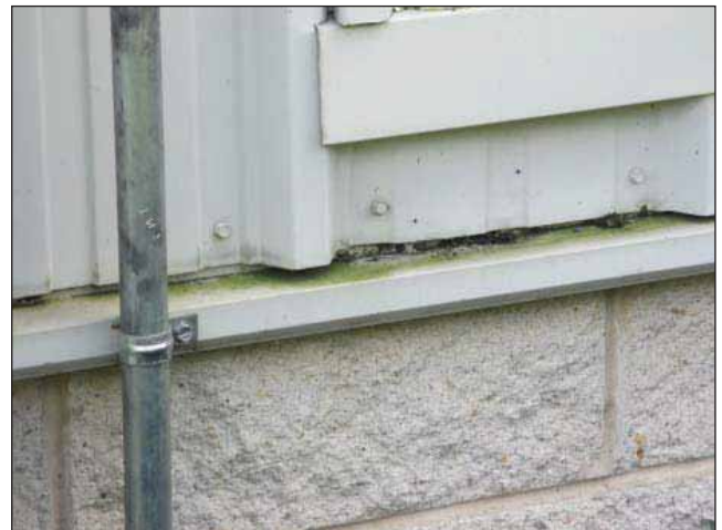
Image 16: Window and frame with molding caused by a lack of proper drainage
