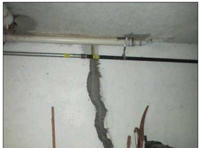
Image 3: Basement with cracking in exterior wall.
