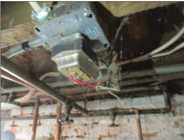
Image 21: Exposed wiring in basement ceiling.
