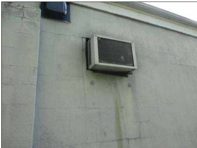
Image 21: HVAC unit has been installed where it appears a previous window was located.
