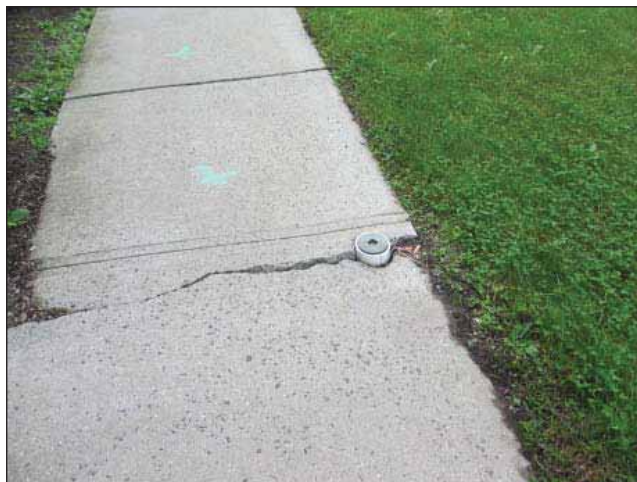
Image 12: Front sidewalk with cracking caused by a lack of proper drainage
