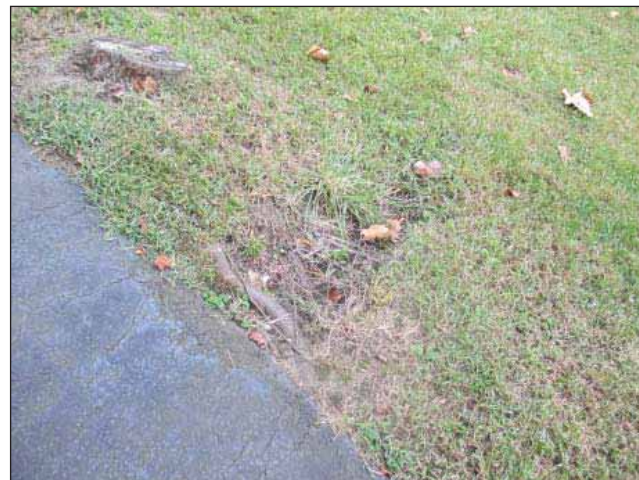
Image 12: Water damage along asphalt sidewalk at rear of the building with erosion.
