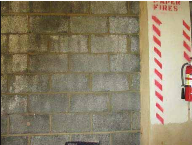
Image 14: Leaching along storage area walls depicting water damage.
