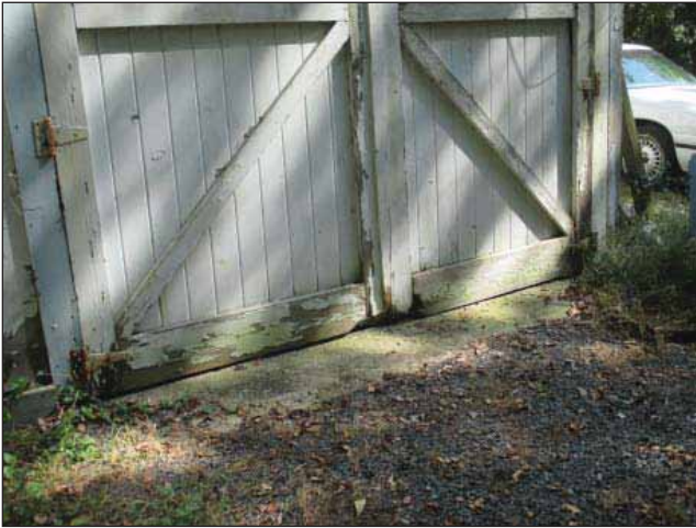
Image 7: Rotting wood along barn door
