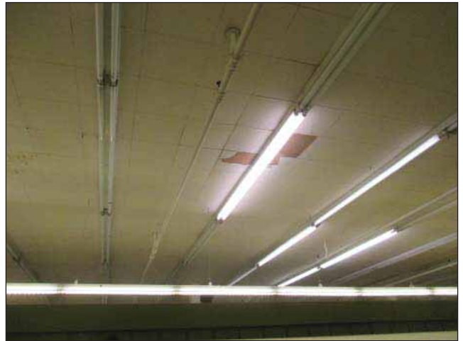
Image 3: Damage on ceiling tiles in the retail area
