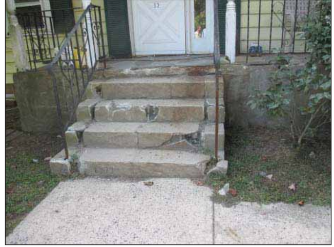
Image 4: Significant deterioration of existing concrete steps to front entrance of the house.
