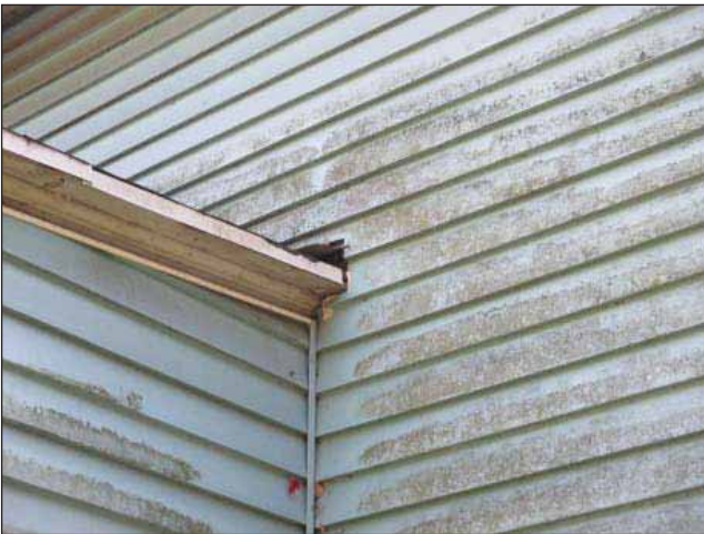
Image 9: Holes at confluence of the side roof and the side siding.
