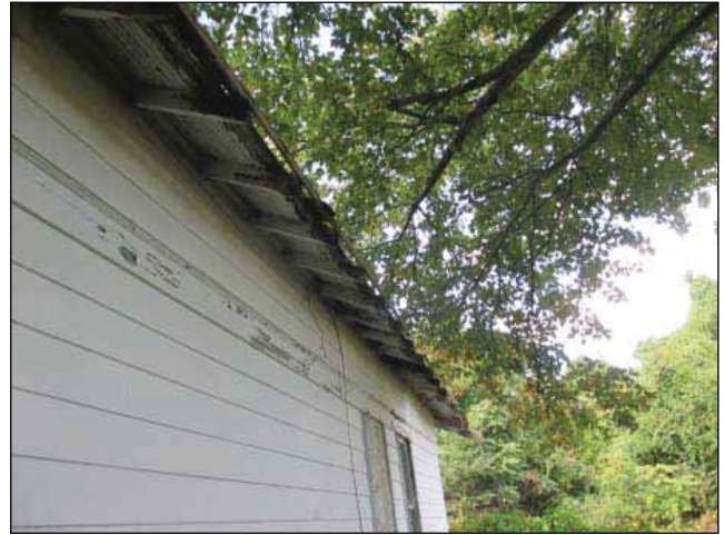
Image 9: Roof completely deteriorated at rear of house.
