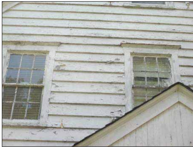
Image 11: Siding damage on two story residential building.
