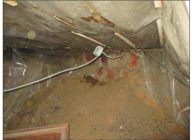
Image 20: Electrical lines hanging in the basement.
