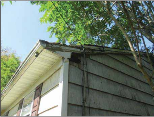
Image 1: Hole in siding to attic space. Rotting wood at roof.
