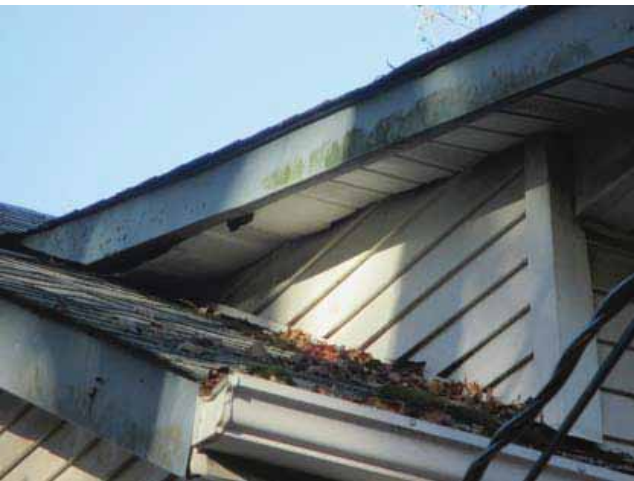
Image 9: Damage to underside of eave.
