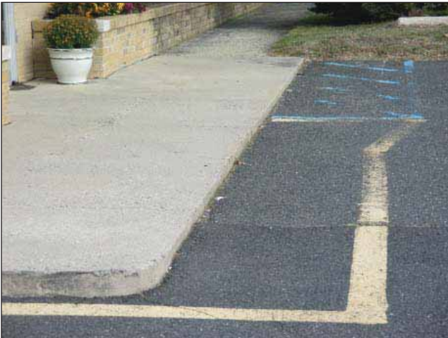
Image 6: Sidewalk at front entrance with handicap spaces which lack proper striping.
