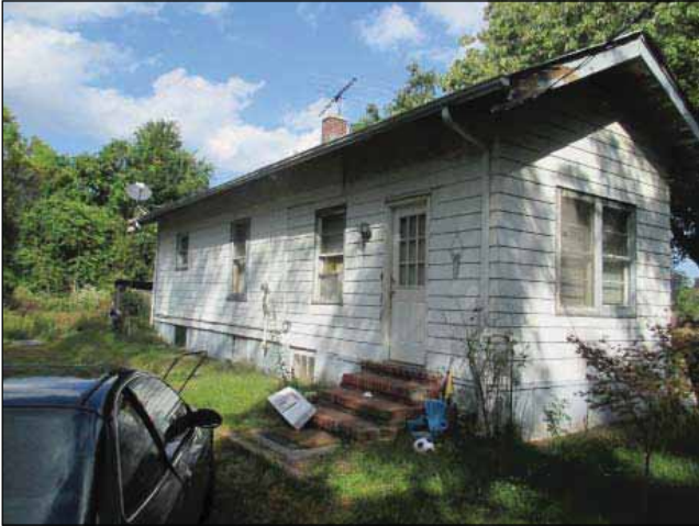
Image 3: Front steps missing hand rails.
