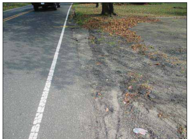
Image 3: Erosion along Kings Highway with no curb and gutter
