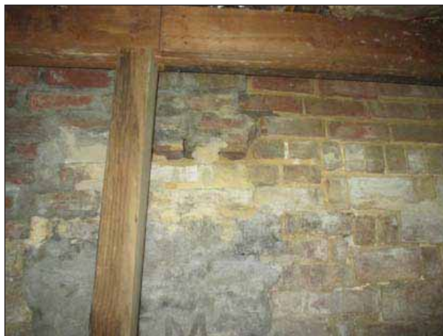
Image 14: Repaired foundation wall in basement with cracking.
