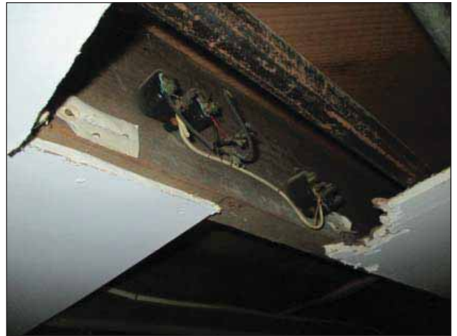
Image 14: Exposed wiring in basement.
