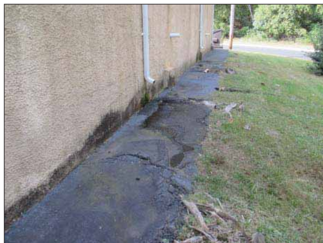
Image 10: Water damage along asphalt sidewalk at rear of the building with erosion.
