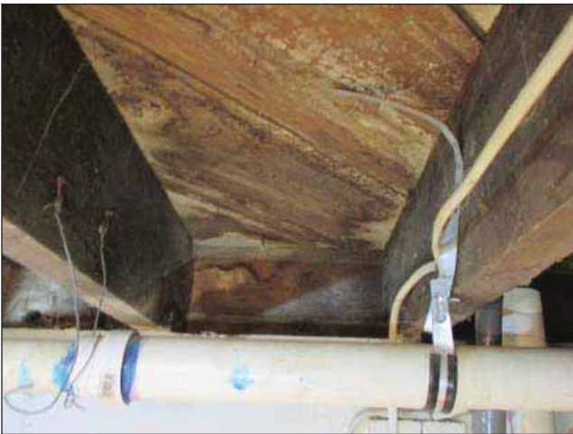
Image 15: Water damage along beams in basement.
