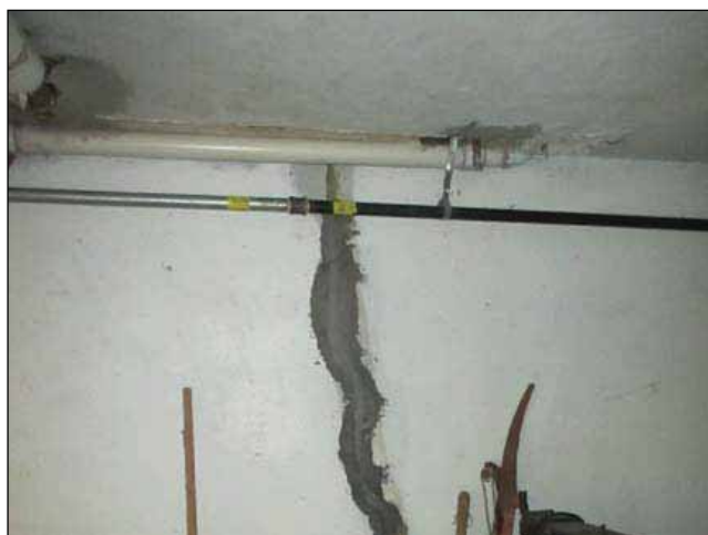
Image 27: Basement with cracking in exterior wall.
