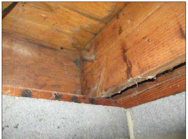
Image 22: Beams of basement with water damage
