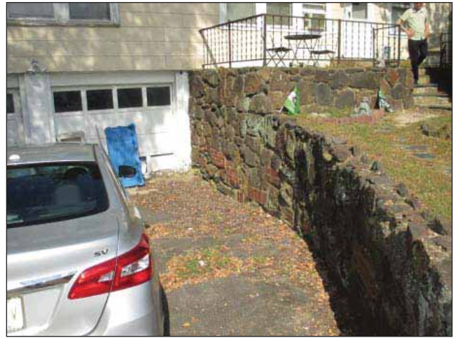
Image 2: Driveway retaining wall with cracking.
