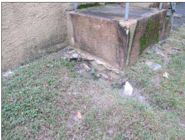
Image 7: Rear stairs with erosion caused by water run-off from roof.
