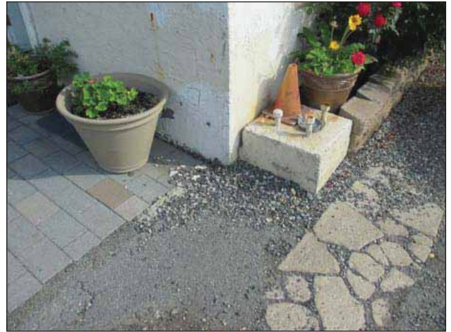
Image 5: Erosion and sediment from rain and run off.
