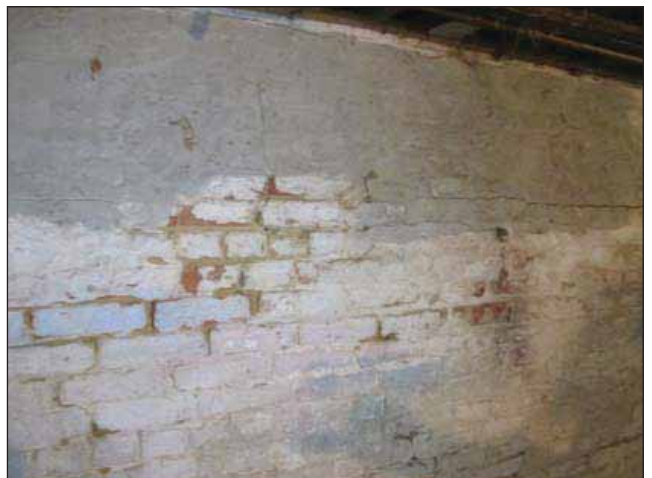
Image 24: Cracks along foundation wall in basement.
