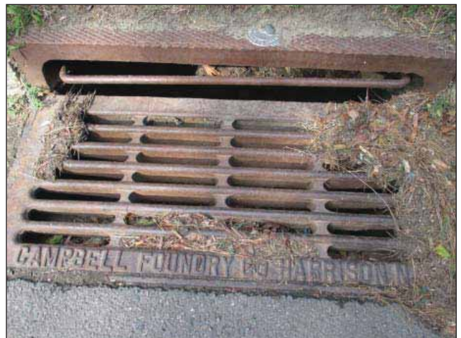
Image 24: Drain inlet with debris
