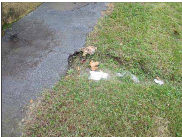
Image 11: Water damage along asphalt sidewalk at rear of the building with erosion.
