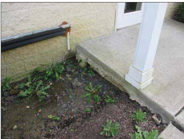
Image 11: Entrance concrete with erosion of the sub-base area most likely caused by a lack of proper drainage
