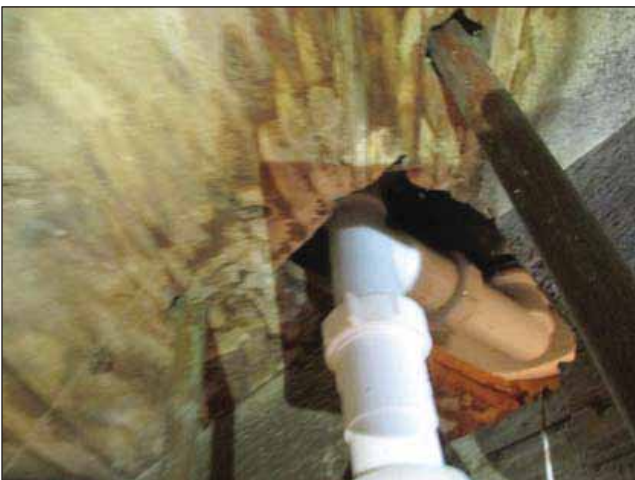
Image 17: Water damage on basement ceiling.
