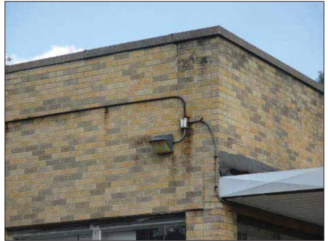
Image 5: Water damage along vertical bricks at roof line.
