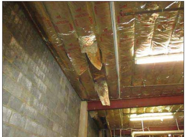
Image 15: Ceiling insulation falling down in storage area.
