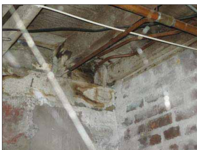
Image 18: Various patching repairs to the foundation walls in the basement.
