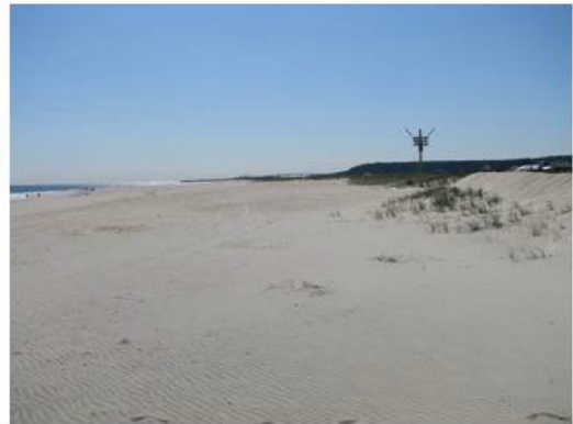
Figure 24. Sand dunes have developed on the former berm following the Monmouth County Federal beach nourishment project. Sand was placed at this location through a cooperative effort between the USACE and US Park Service in 2002. (Left photo January 10, 1995 [view to the southeast]; right photo October 6, 2011 [view to the south]).
