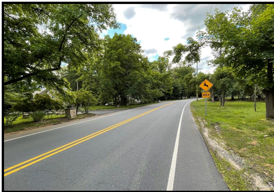
Figure 3: Sight Distance limitations at the West Nut Swamp Road and Crawfords Corner Road intersection. View from southbound approach on Crawfords Corner Road. (Photo taken by T&M on May 29, 2024)
