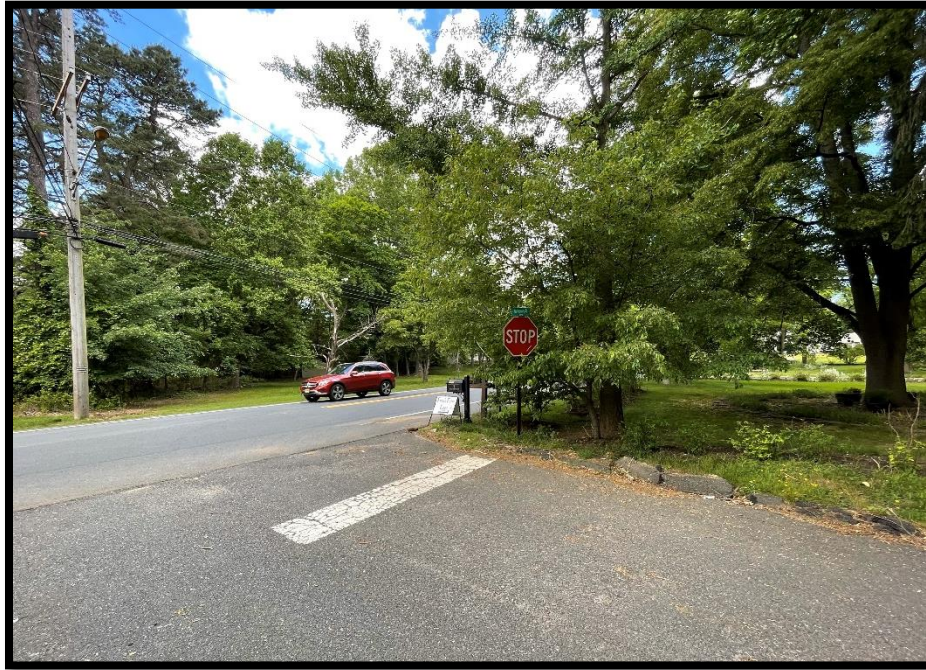
Figure 2: Sight Distance limitations at the West Nut Swamp Road and Crawfords Corner Road intersection. View from the West Nut Swamp Road approach. (Photo taken by T&M on May 29, 2024)A
