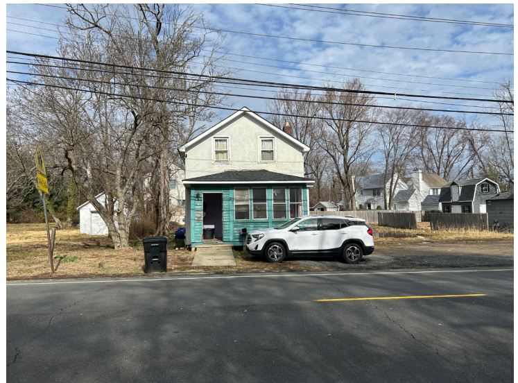
Figure 69: Photo showing the dwelling on Lot 13, showing the missing front door and peeling paint.
