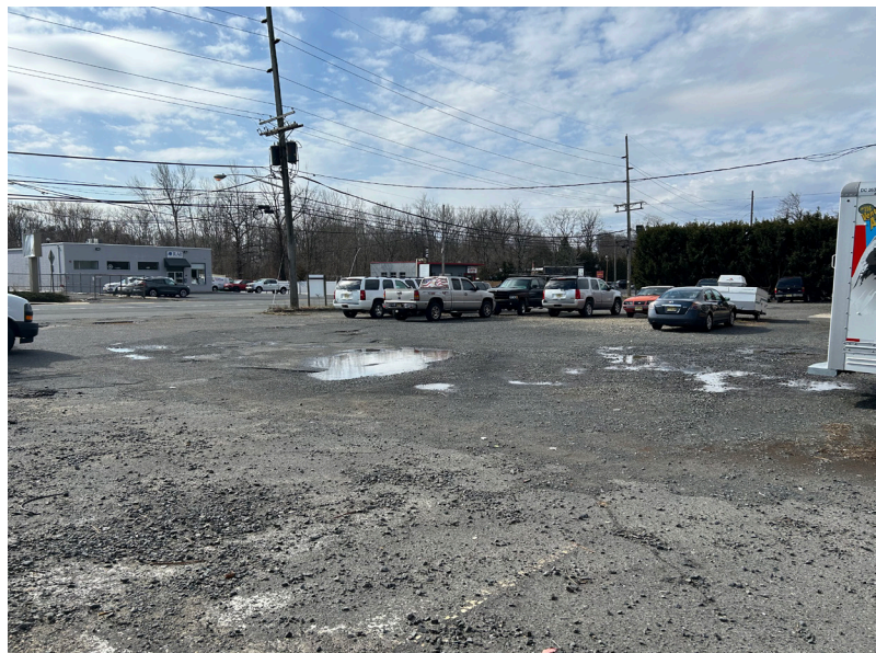
Figure 54: Photo illustrating the parking lot and drainage issues.
