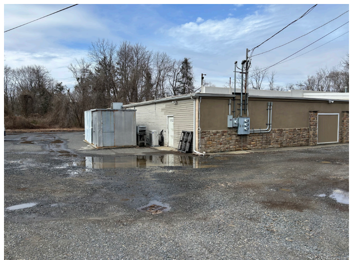
Figure 94: Photo showing the rear of the building on Lot 27, along with the drainage issues observed.
