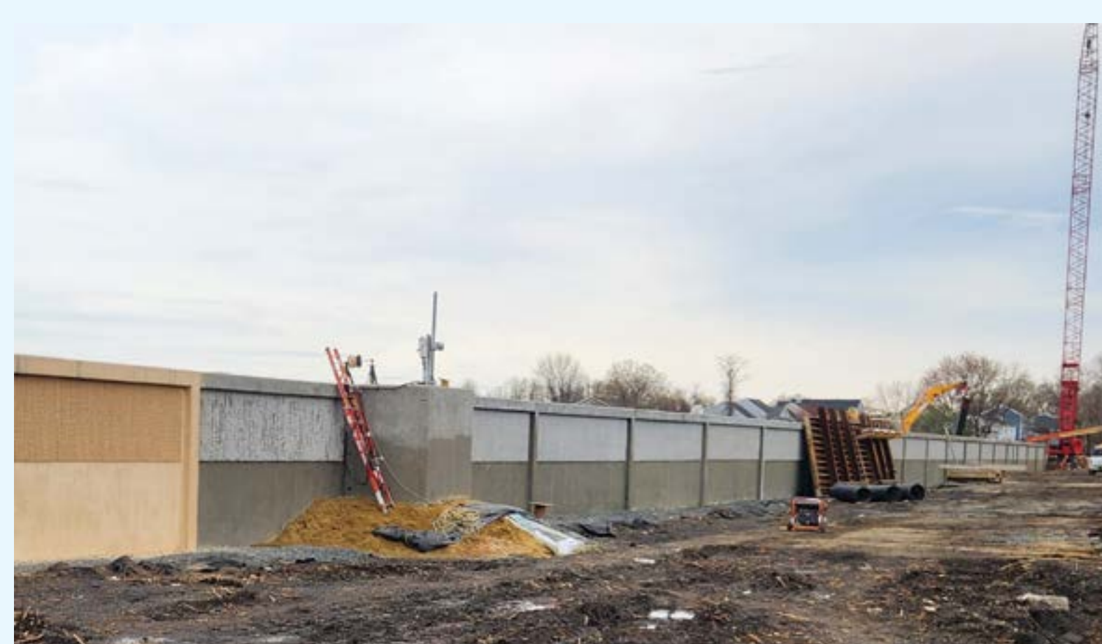
The construction of a new concrete floodwall continues along Main Street in Port Monmouth.
