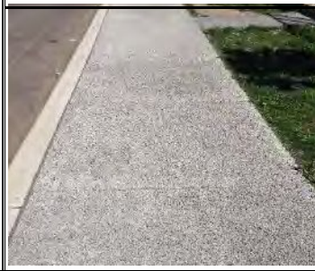
Permeable Pavement (Camden, NJ)
