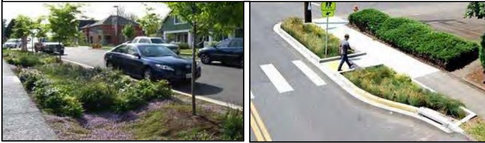
Bioswales (Source: EPA)
